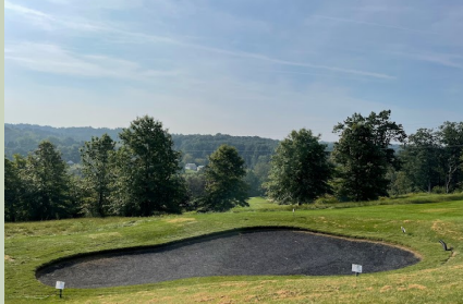
New fairway bunker on 12 showing the liner (Blinder) and edge structure (EcoBunker)
